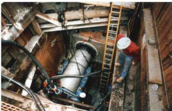
Figure 2- Typical pipe arrangement at the driving end/shaft of micro tunnelling
