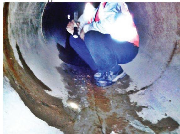
Figure 4 - Cracking of polycrete pipes
